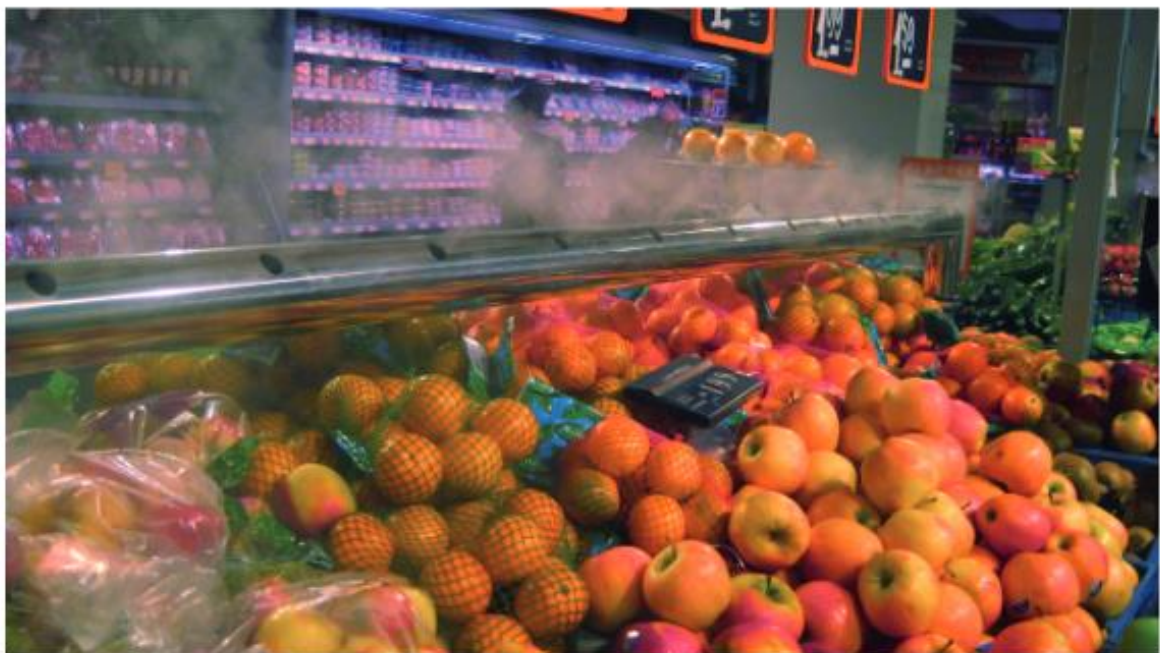
Figure 2: Humidification of fruit and vegetables in a supermarket
