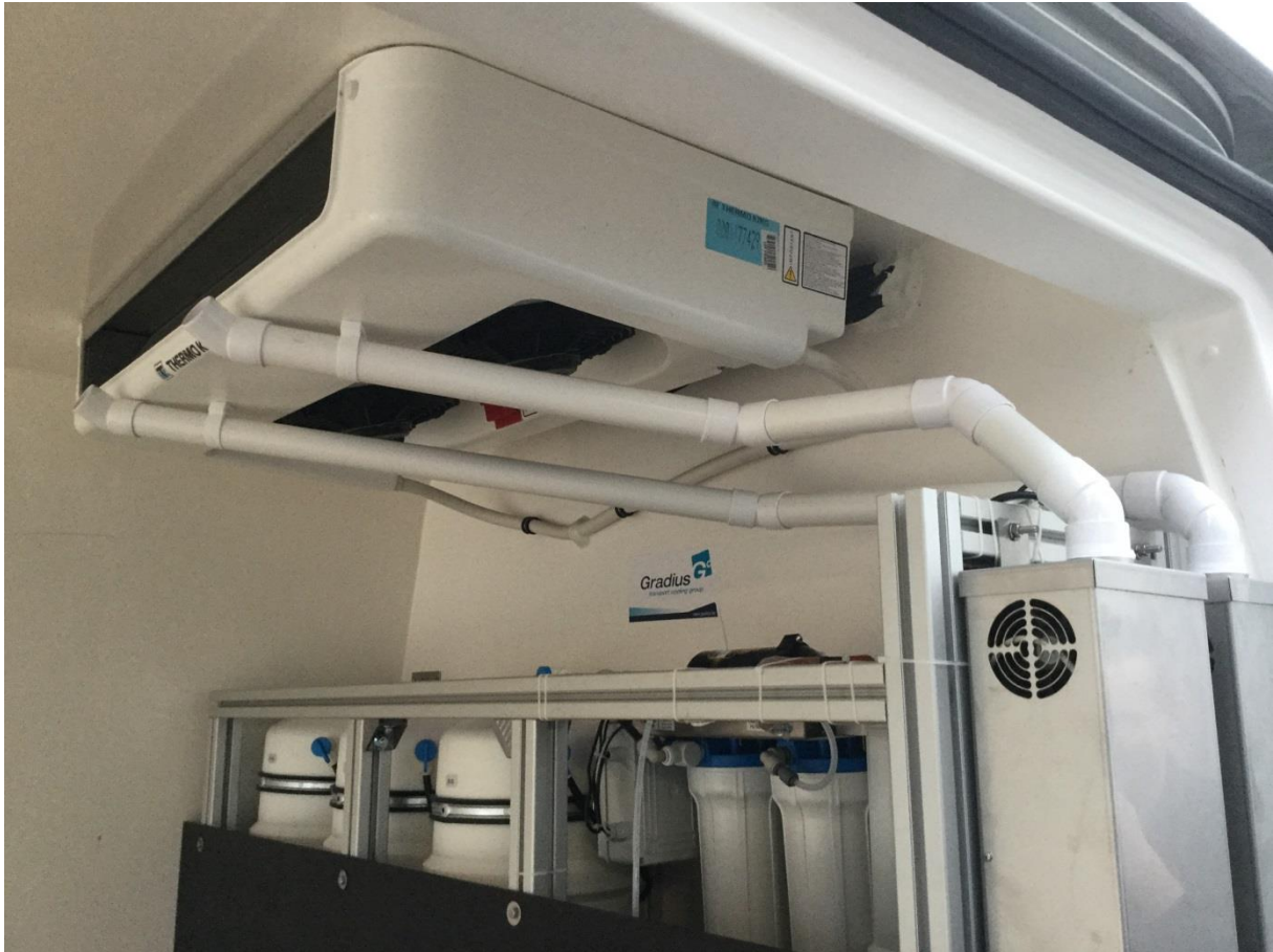
Figure 11: 2 Mobile humidifiers with outlets and cooling unit in the Van
