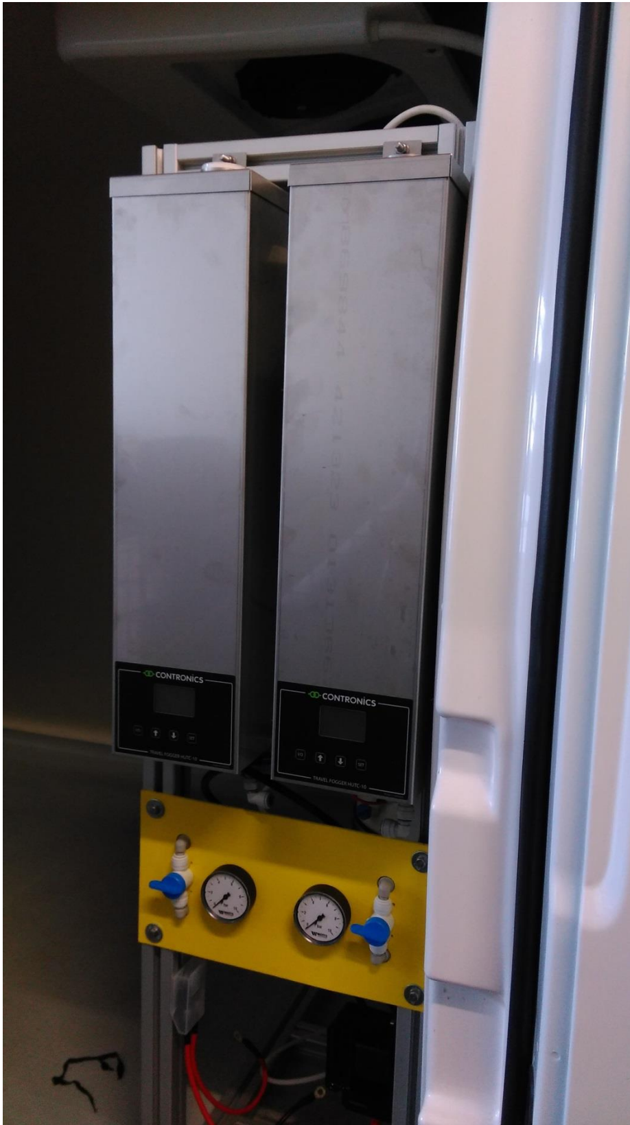
Figure 10: 2 Mobile humidifiers installed in the Van
